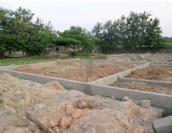
The foundation walls
